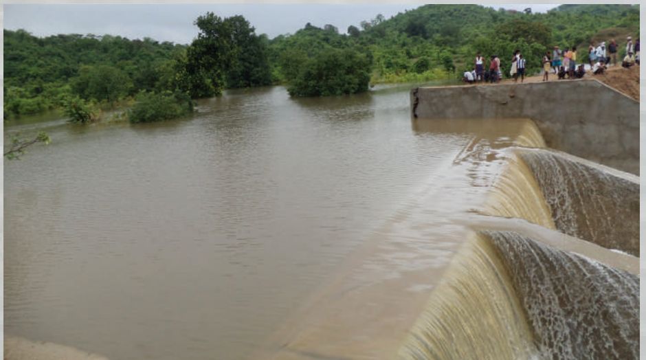
The image of the water conserved for about 3 kilometers behind the dam after the construction of Budha-Budhi Dam. This is the same place where not even a single drop of water coming from the hills in the form of rainwater stayed.
